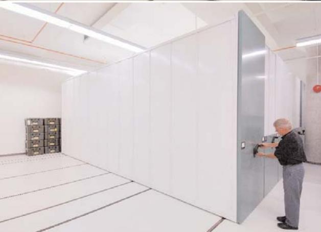
The mobile system in the Living History Vault, which is a cross-section of all other vaults, had to be securable due to its small firearms collection. It was designed as a self-sealing system, which compresses against one wall, with lockable end unit to comply with the Canadian Fire Arms Act. Compact mobile systems also saved footprint space in the 3D Map Archives, Photo Archives, Paper Archives and Research Library.
