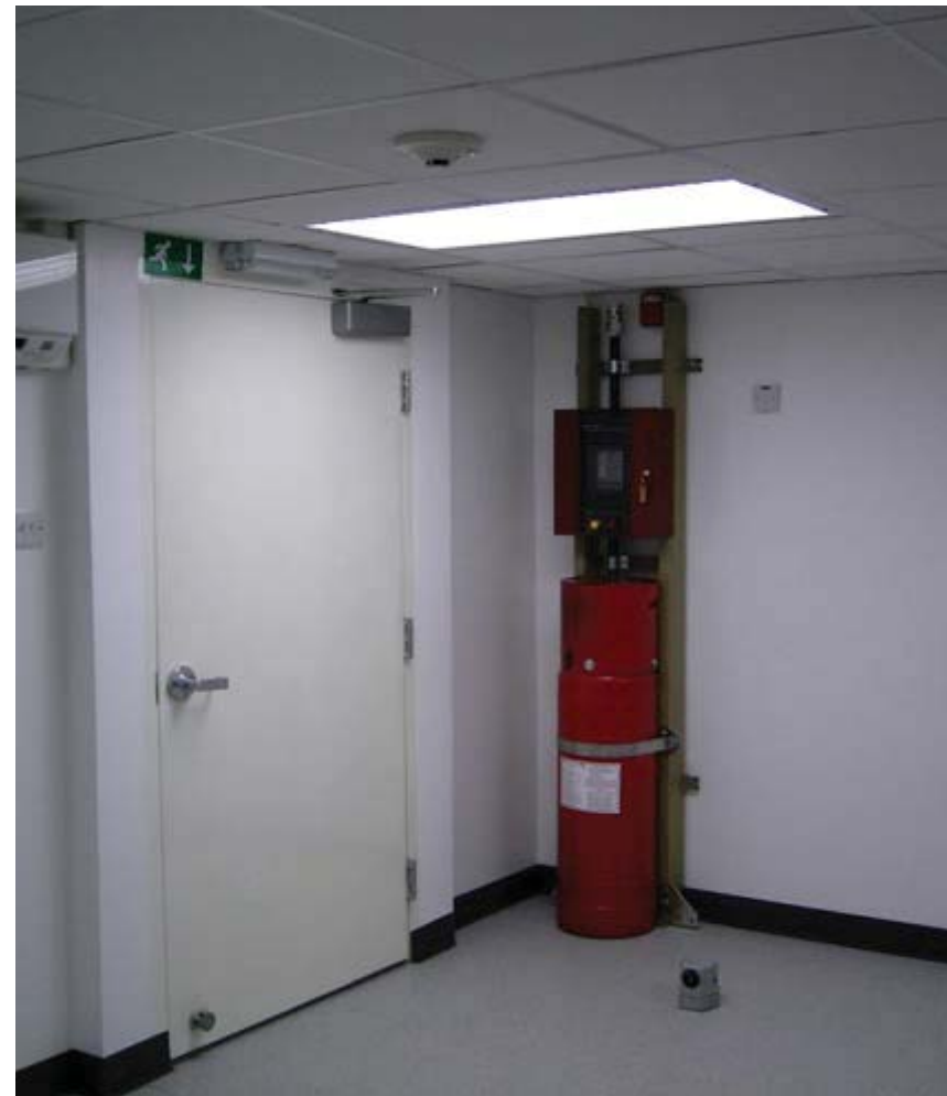
Inner Vault Door for Media Protection & Clean Agent System
