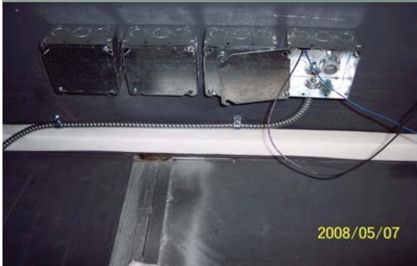
Cable Tray on vault Roof & Inner Electrical Boxes for Vault Service
