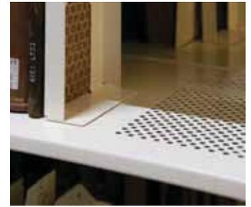
Perforation helps eliminate stratification of highly filtered air – and allows for more precise environmental control. It also boosts the circulation of a clean-agent mist, and aids in extremely early detection of a potential fire.
